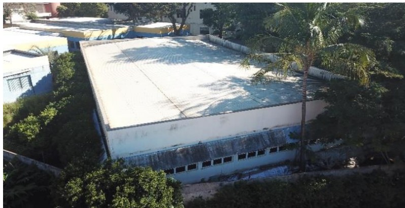
Figure 3. Right Side (SE) of the Library.
